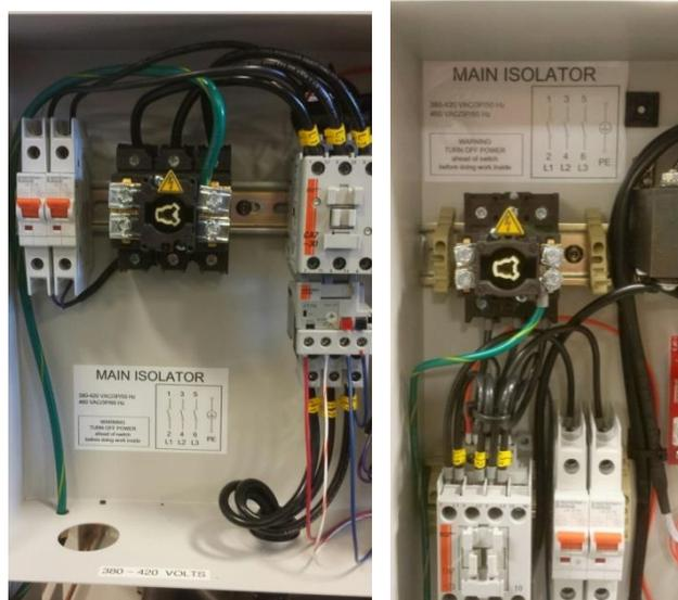
Figure 3-11, Main Isolator Wiring
