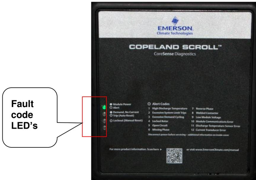
Figure 5-3, Emerson Compressor Front Panel Fault Code LED's
