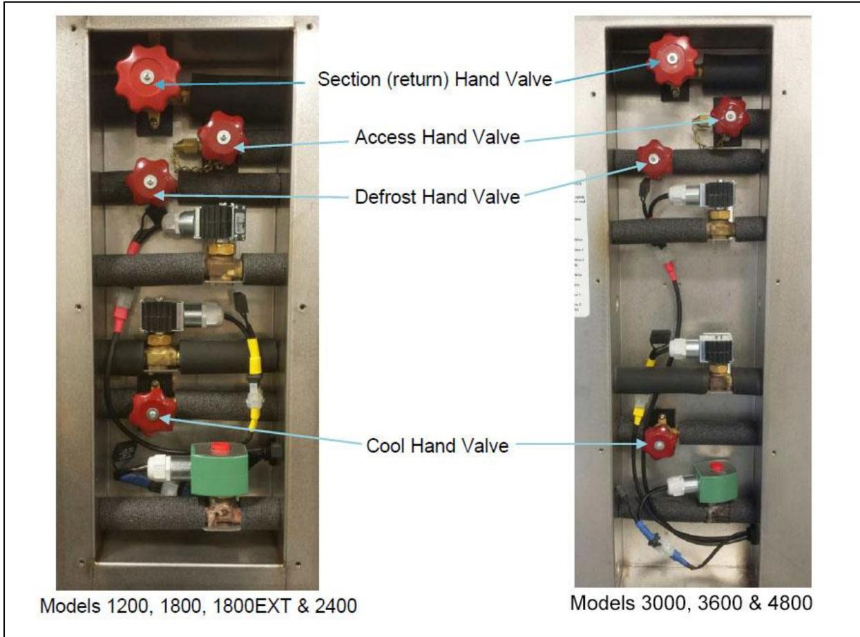
Figure 3-5, Position of Hand Valves
